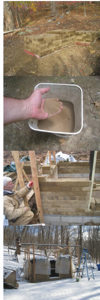
From above: The bricks stacked on palettes; "Brown sugar" used for the slurry instead of mortar; setting the bricks in place - note how they would dry once they were set and exposed to air; the shed project survived a winter.
