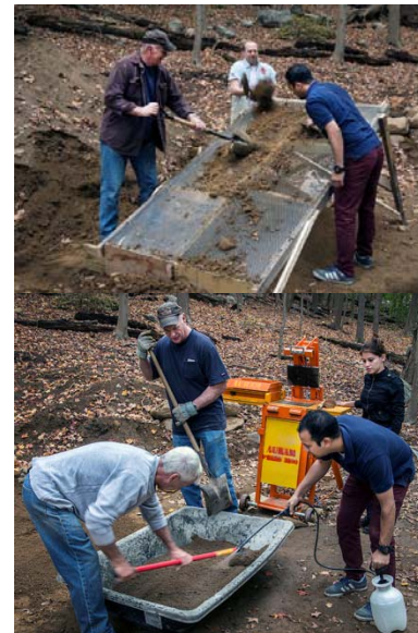
Screening the dirt pile above; mixing the soil, Portland Cement and water below; Photos by Philip Jensen-Carter
